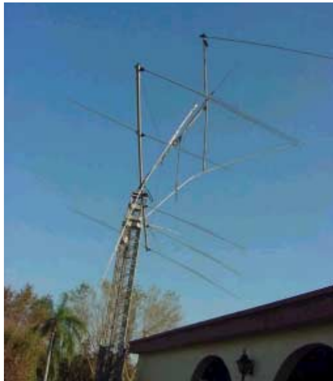
N8PR - Hollywood One Tower and Antennas
