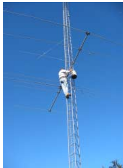
Dan K1TO works to raise the C3 to the top of his new 160 foot tower
