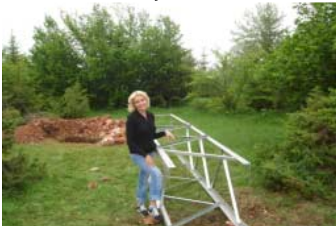
Danny's wife Viki helps with assembly of the first tower section
