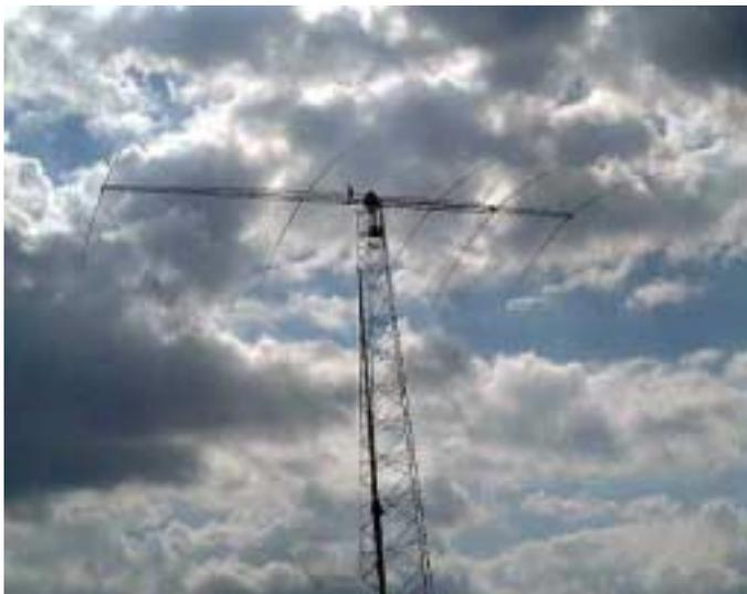
*FCGers wondering what to do for added effectiveness on 80 meters this season might want to consider one of the above! It's a 5 element array in use at 7J4ARL. Construction was supervised by JA4UEP. It was finished October 19. The small dot on the boom left of the tower top may be a worker, perhaps JA4UEP himself! (Tnx Bill K4XS for bringing this monster antenna to our attention).*
